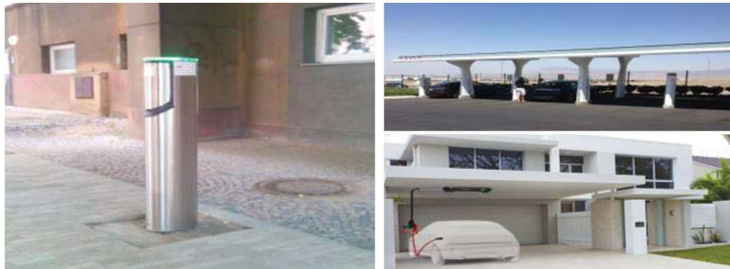
Figure 1. Examples of EV charging stations: corporate station at Transportation Faculty, CTU in Prague (left), Tesla public charging station with solar energy source (upper right), home charge station by Easy charge (bottom right)
