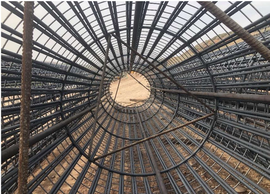
Figure 3. Reinforcement cage
